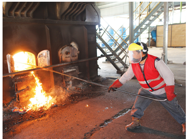
Boiler handler at PTNJL
